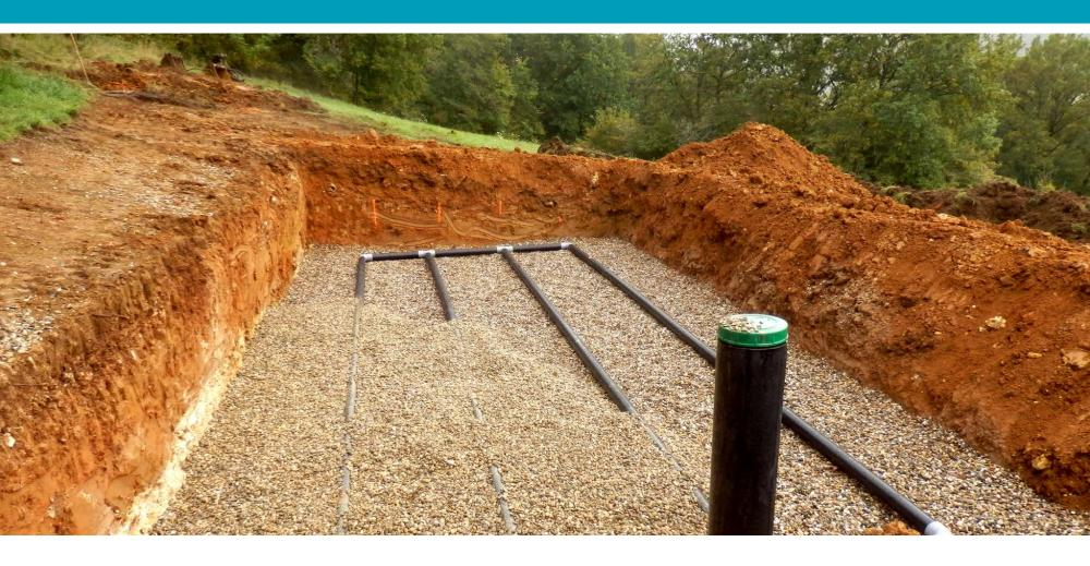
The size of the septic system is determined by engineers and is based on the number of bedrooms in a house rather than the size of a home. The number of people living in a home is important in determining the parameters of the system. The more people, the larger the system because there will be greater demand for it to process wastewater from toilet use, showers, dish washing, laundry, and so on.
